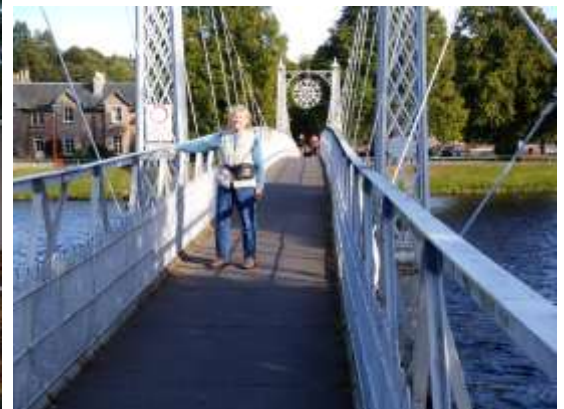
A decorative bridge across the River Ness
